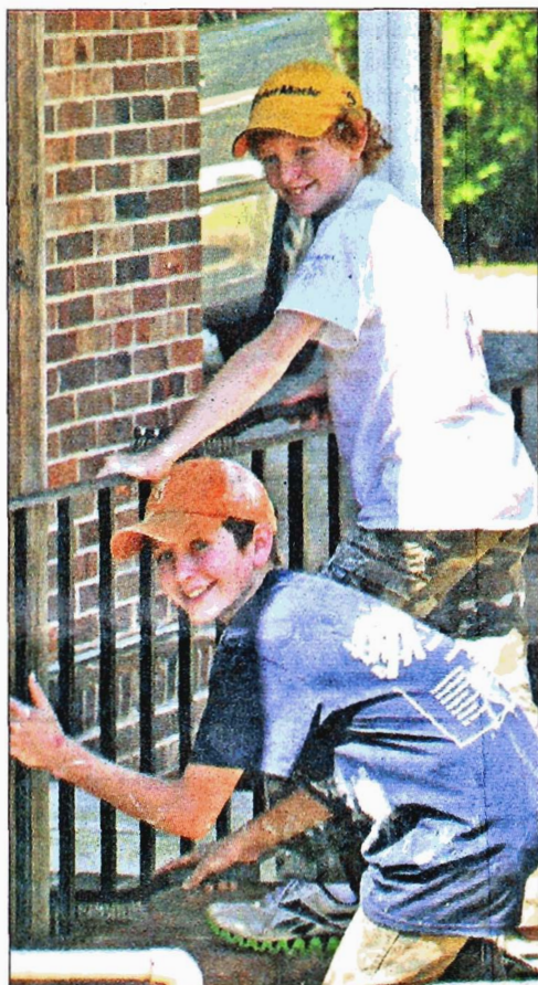
Browning Sandusky and Scooter Barnes scrape all the rust off these hand rails in preparation for repainting them.
